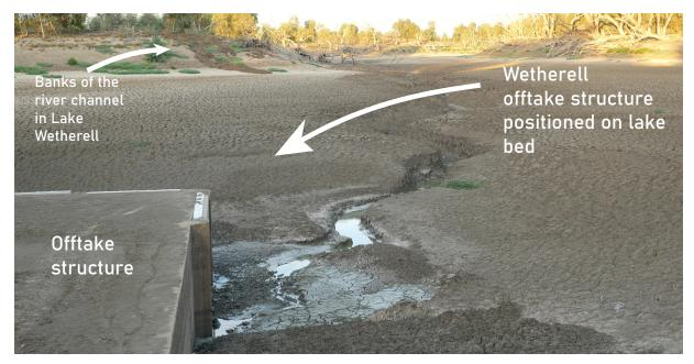
Figure 15 - Lake Wetherell pictured March 2020. Offtake structure draws water from the bottom of the lake bed. Photo by Dan Schulz on March 11, 2020
