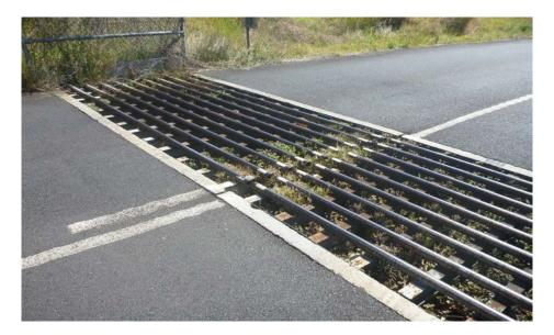
Fig 2. Example of proposed koala roller grids to be installed
