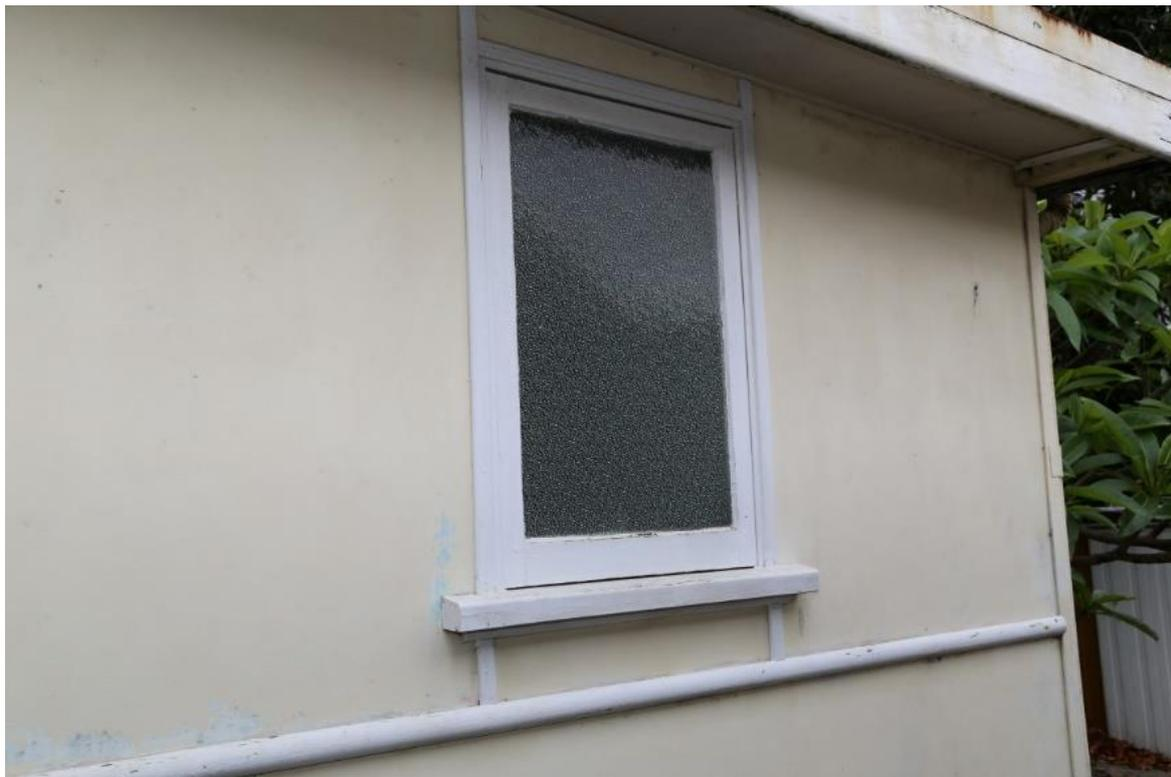
**Figure 3.4: Bonded asbestos cement sheeting**
